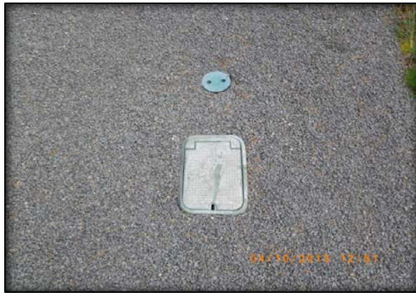
Picture of new customer valve & AMR after being installed.
