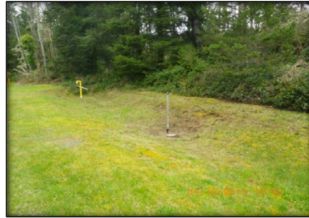
New Standpipe we installed for the middle tank at the NWF.
