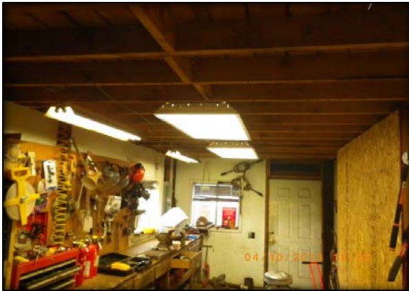
Picture of two more light fixtures that were installed.
