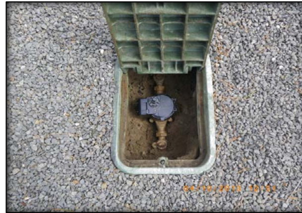
Picture of the new AMR meter after it was installed.
