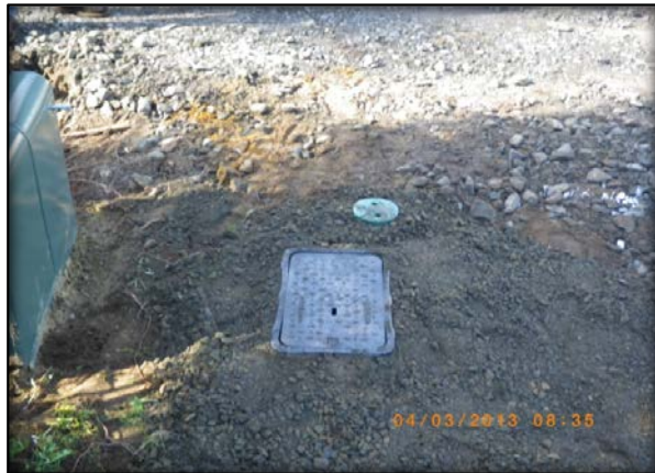
After new service was installed.
