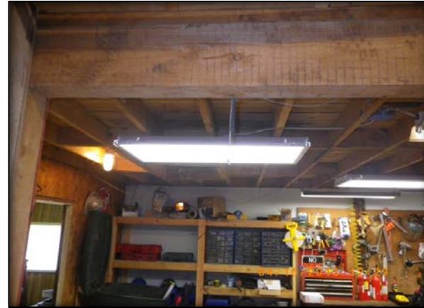
New light fixture installed in the shop.
