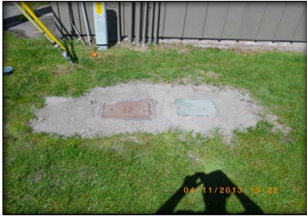
Picture after check valve was installed for Ocean Aire Trailer Park.
