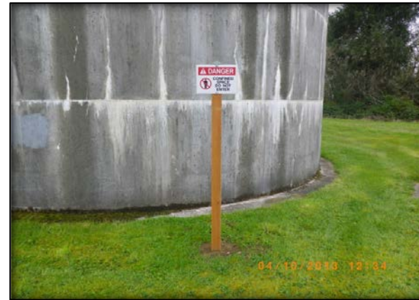
The new confined space signs we put in next to all four reservoirs.
