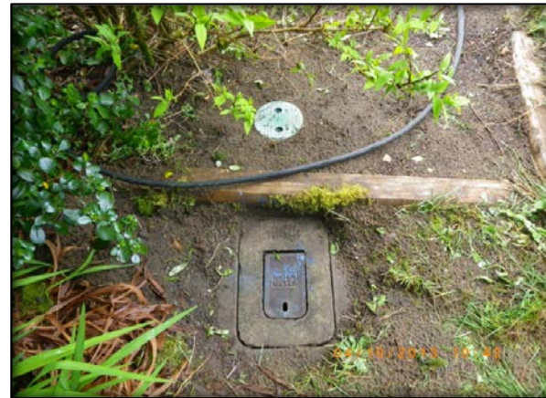
Picture of after Customer valve was installed.
