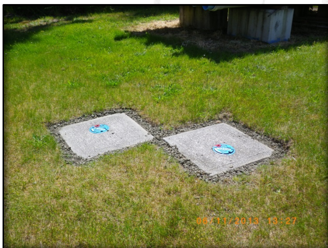
Picture of the valve slabs touched up.
