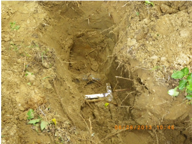
Service tap for the customer's service.
