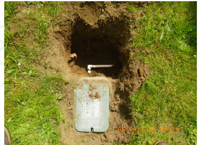
After customers water line was dug up.
