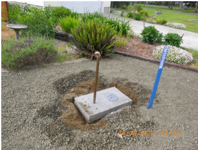
New standpipe down 194 th Ln
