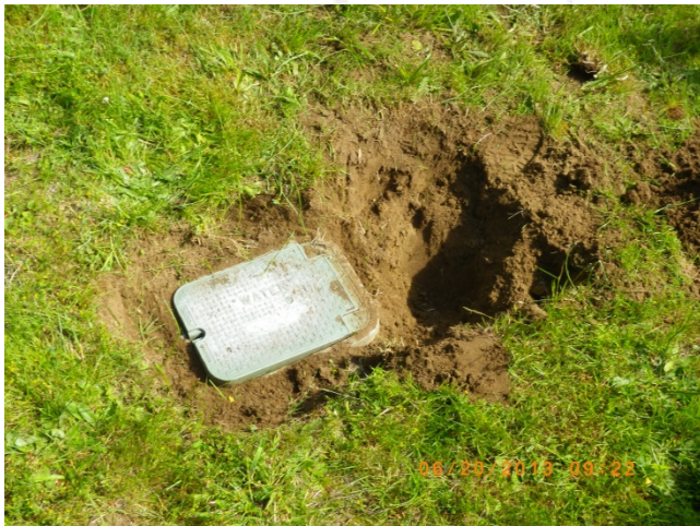
Before customer valve installation.
