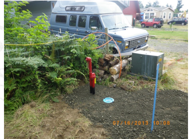
After new blow off was installed.
