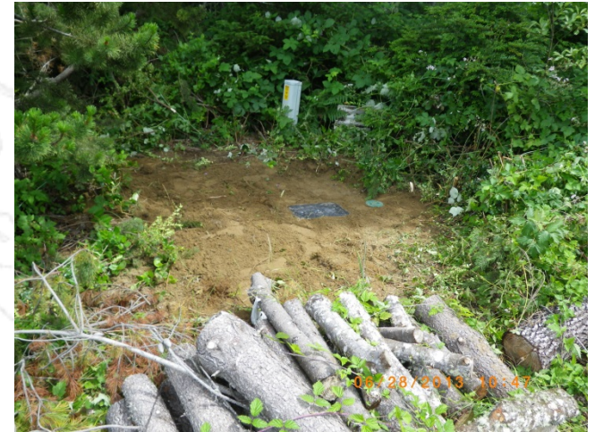
After the new service was installed.
