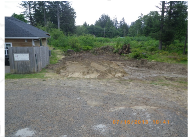
Picture of after we finished the restoration where we had a main break.
