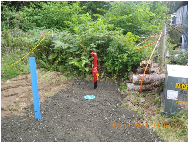
After new blow off was installed
