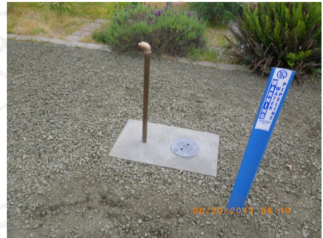
New standpipe after the gravel was raked back.
