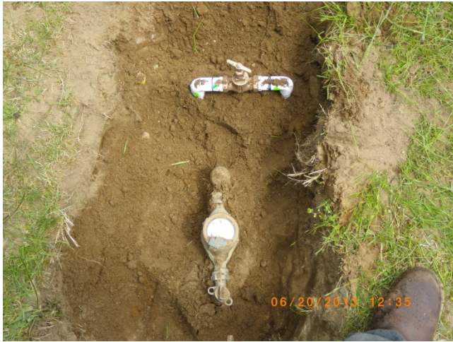
Picture of customer's valve installed.
