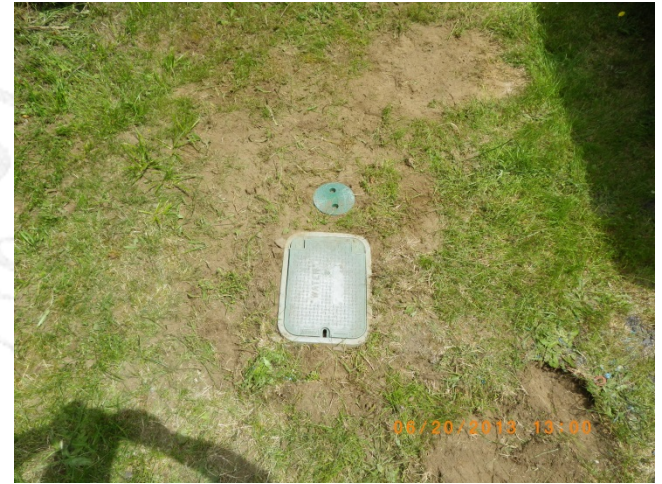
After the customer's valve was installed.
