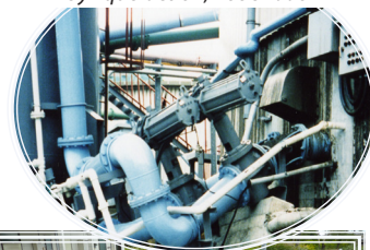
Higashinada WWTP ravaged by liquefaction, Kobe 1995
