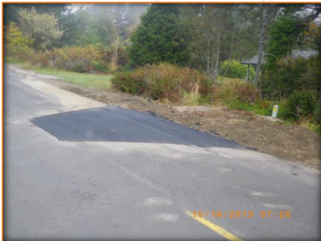
After the road was restored from the leak on 274 th .
