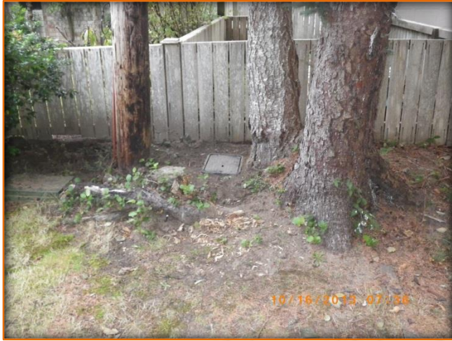
Picture of a meter box replacement.
