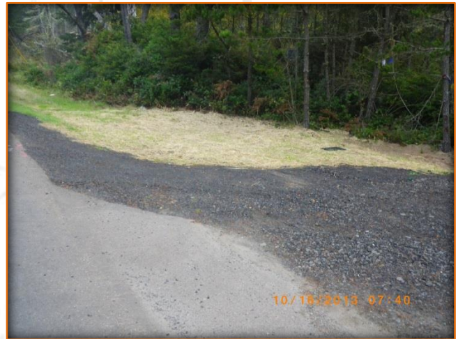
Picture of the new service on the highway, along with the road restoration.
