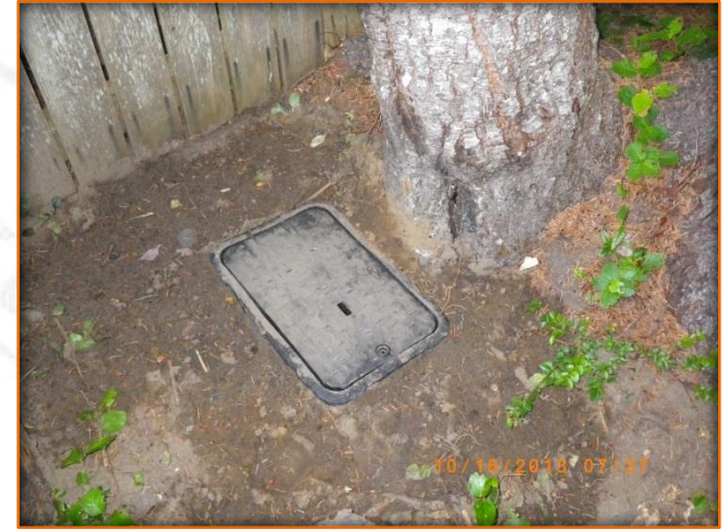
Another picture of a meter box replacement.
