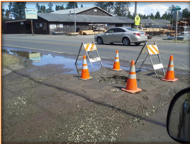
Main Break on 254 th and Vernon.
