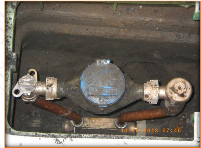
Picture of a new resetter that was installed for Taft plumbing.
