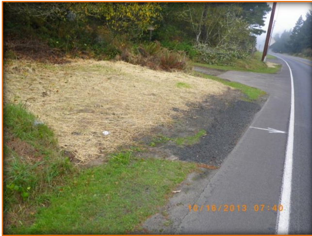
Picture of where we did the tap for the new service and the road restoration.
