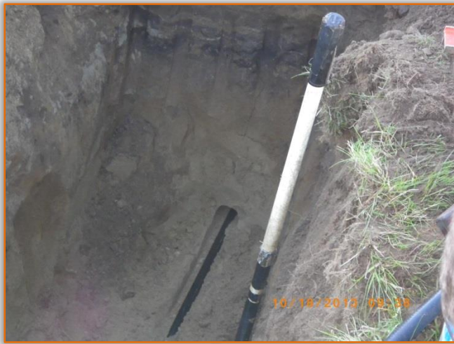
Picture of the mole starting to push across 269 th Pl. for the service re location.
