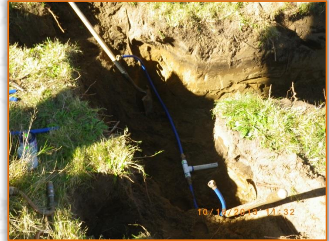
The Service lines for each meter.
