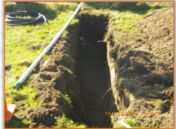
The ditch where the mole will push to.
