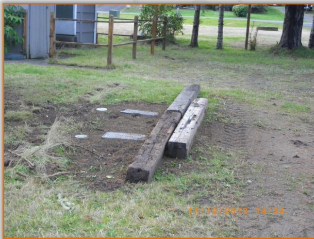
After the two services were re located.
