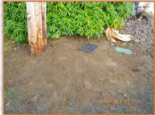
Meter box replacement.
