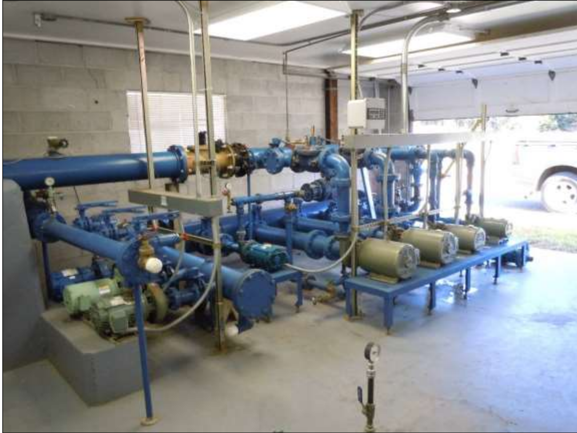
North Well Field Booster Pump Station
