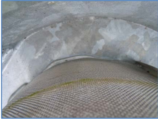
Figure 7 NWF #3 Vent - Side View
