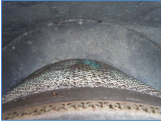
Figure 1 NWE #1 Vent Side View
