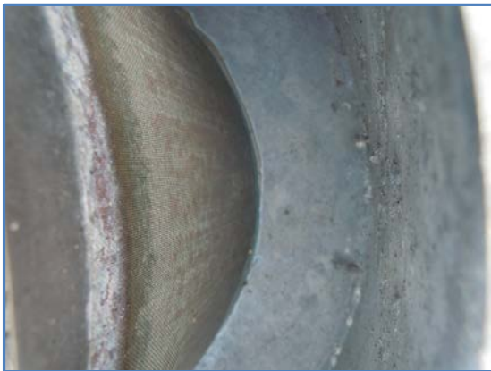
Figure 6 NWF #2 Vent - Side View
