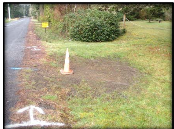
Restoration after repair
