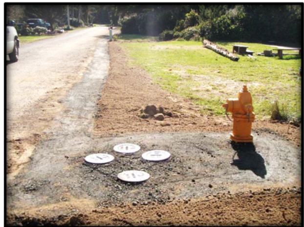
New Fire Hydrant-West side of N Place at the intersection of 308 th Place
