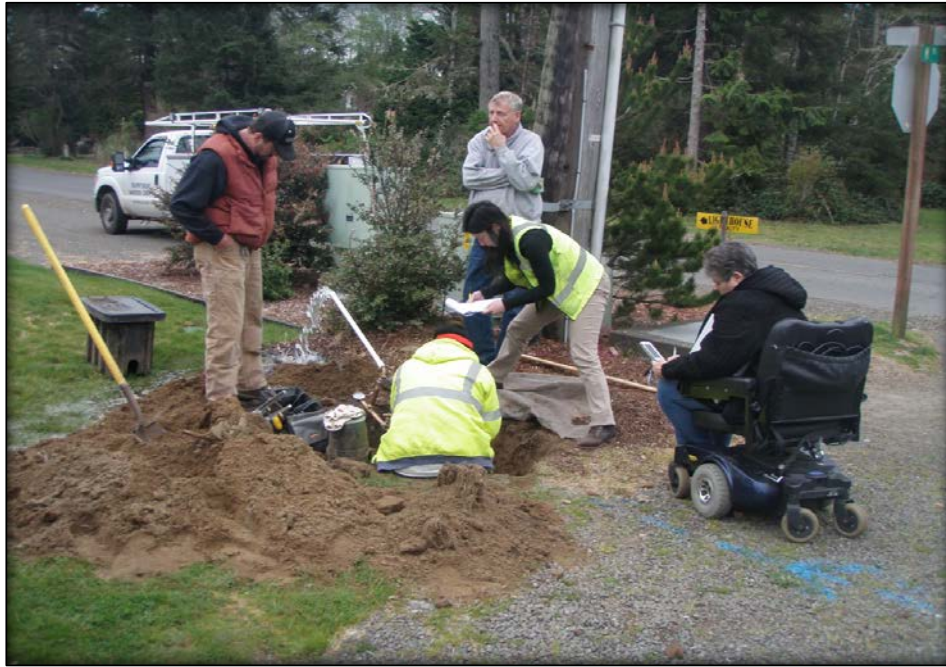
Working with a member to increase flow to sprinkler system.
