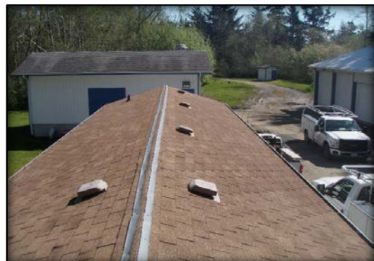
Inspecting Roof (Booster BLDG.)
