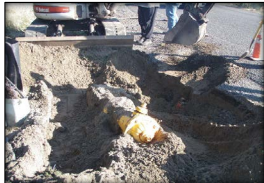
Repairing Fire Hydrant (Hit and Run)
