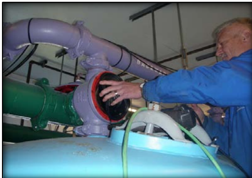
Maintainance on Filter Plant
