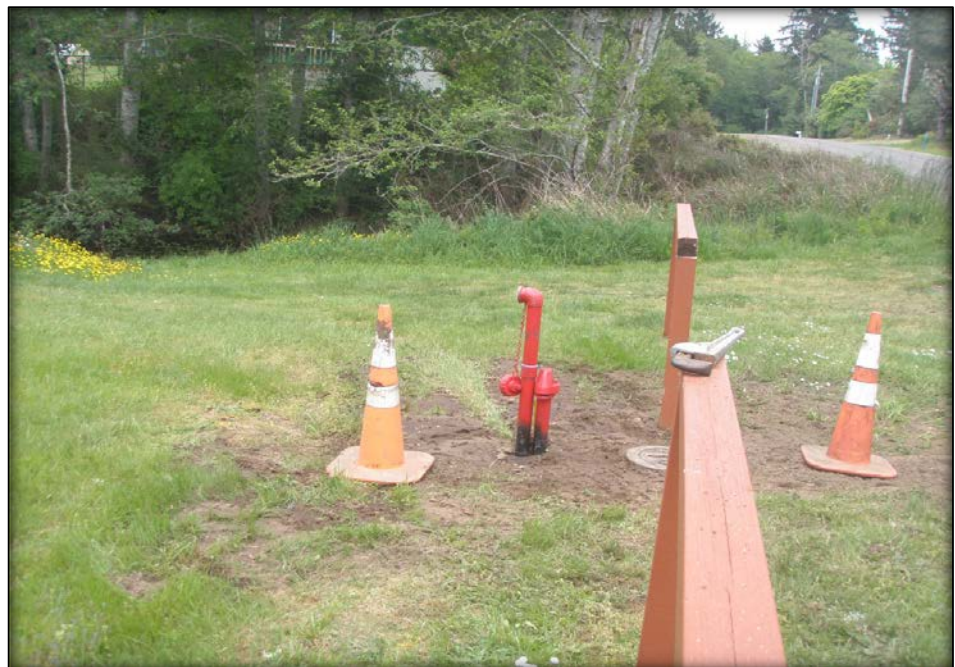
A new flushing station at the Skating Lake Cabana
