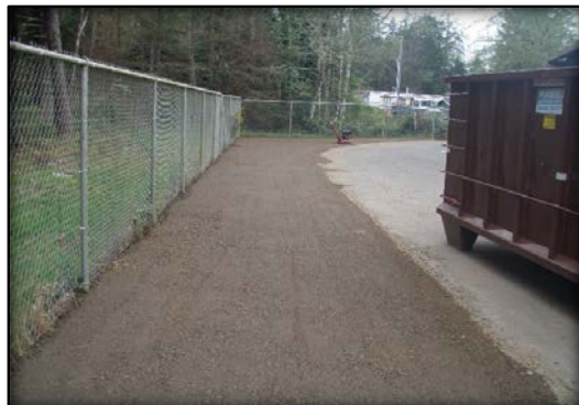
Work at Compactor
