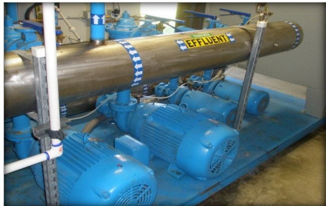
South Wellfield Booster Station
