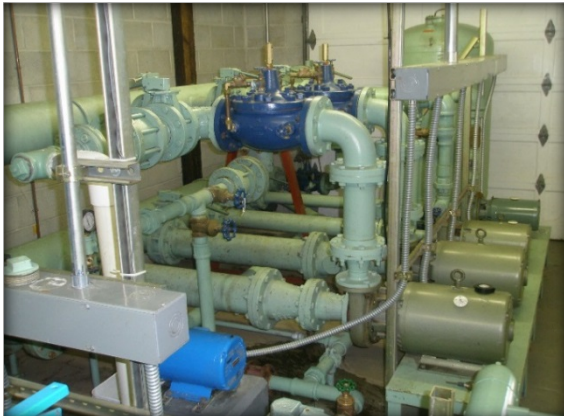
North Wellfield Booster Station
