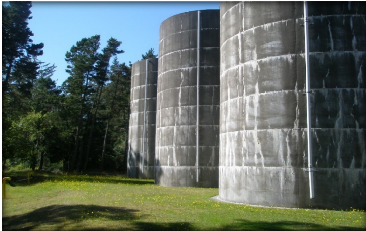
North Wellfield Reservoirs
