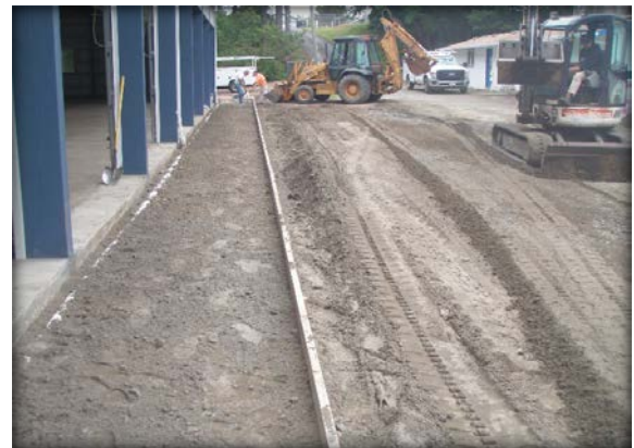
Forming the apron and sidewalks for concrete
