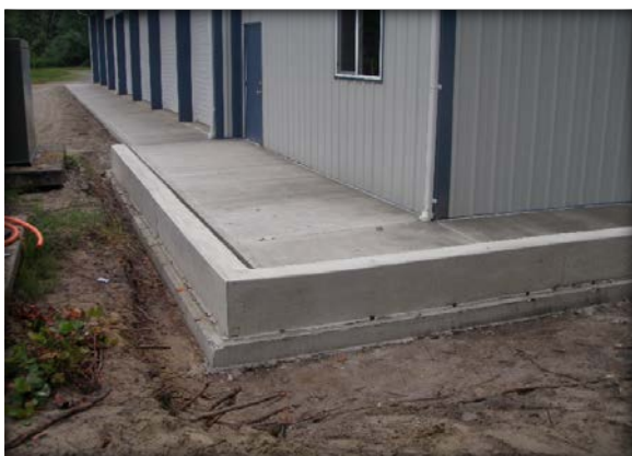
Finished apron and sidewalks
