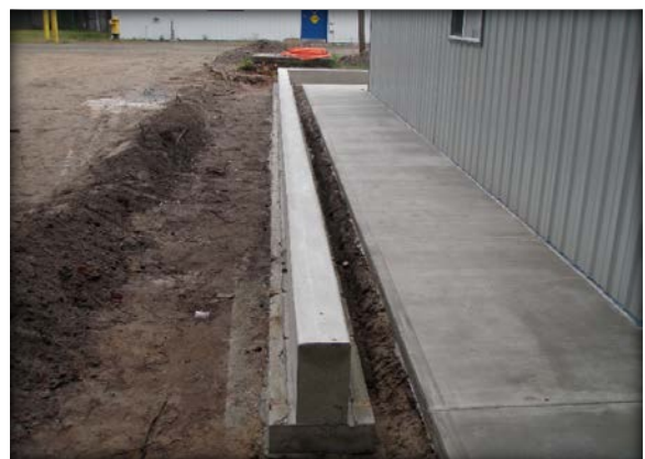
Finished apron and sidewalks
