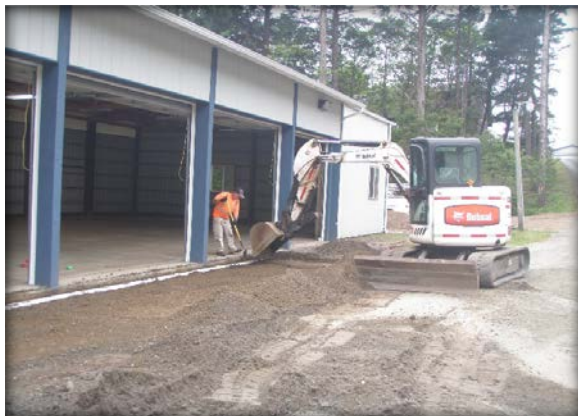
Forming the apron and sidewalks for concrete
