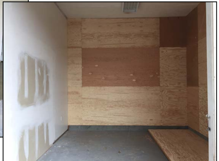
Ferric Room Framed
