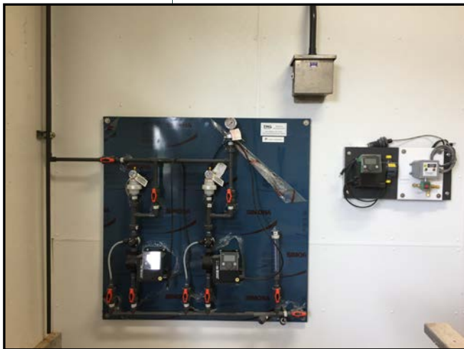
Feed Pumps for Ferric Chloride & Potassium Permanganate
