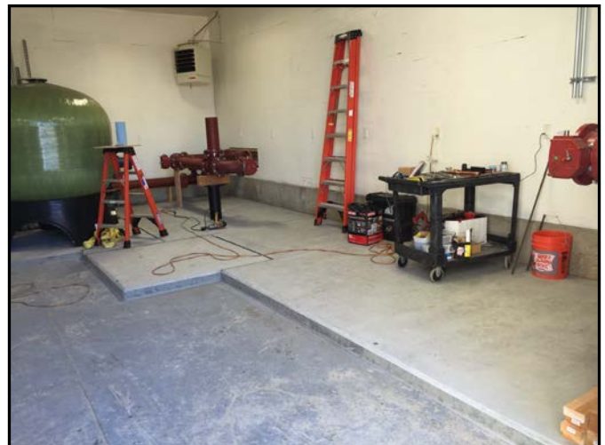
Slab to reinforce concrete floor
