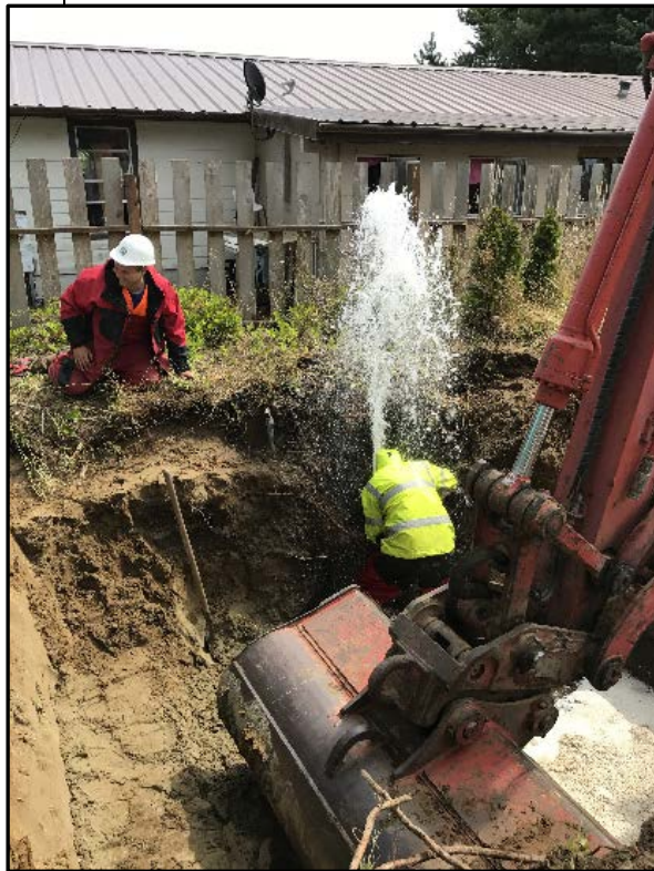
Repairing Main Break. Rushlight Estates
