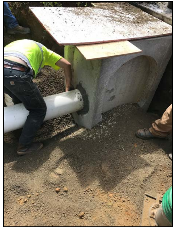
Installing Catch Basin at the SWF Backwash Pond
