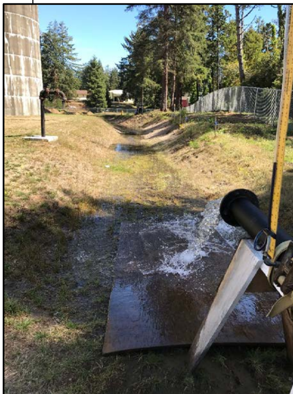
Pump Testing Well #7b (150 GPM)
