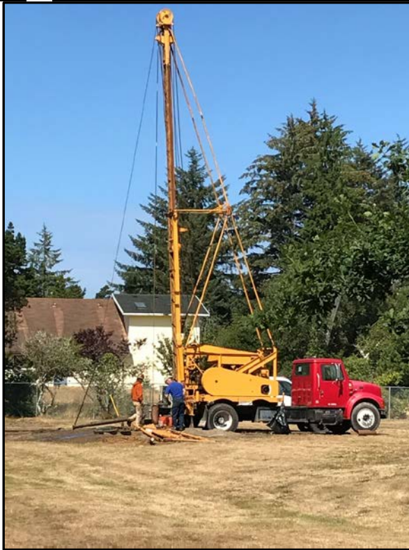
Work on Well #6
