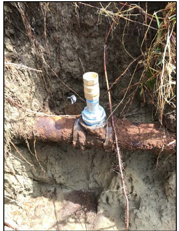
Repairing Main Break. Rushlight Estates
