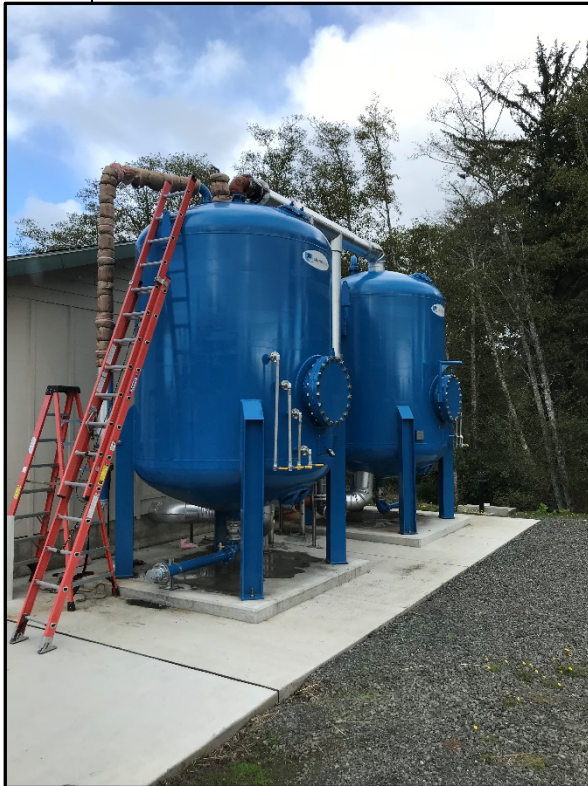
SWF Carbon Filter Vessels
