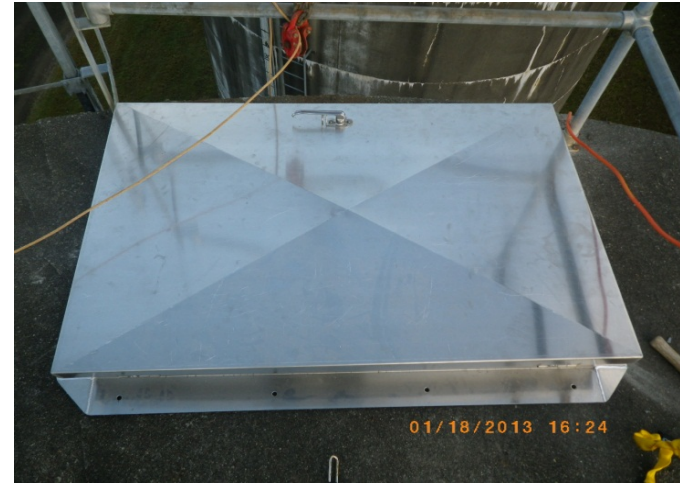
Picture of the new hatch in place.
