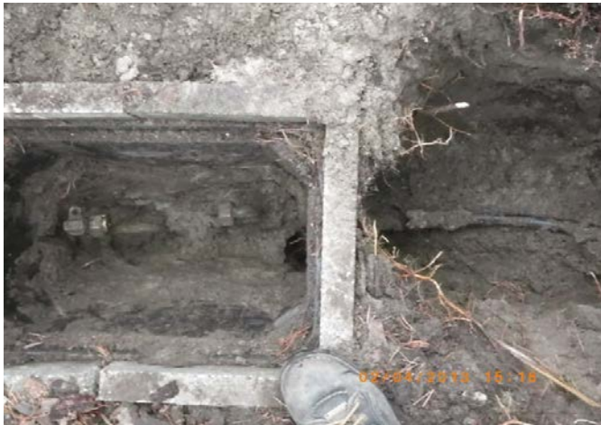
Picture of us working on installing customers valve.
