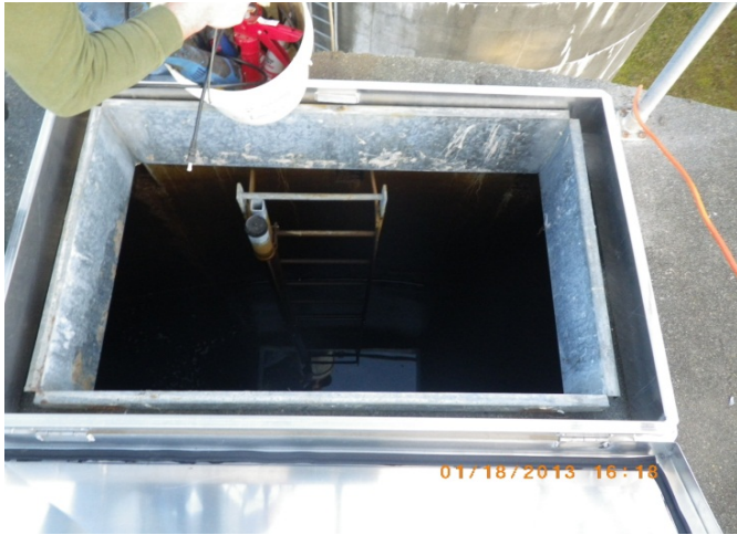
Working on installing the new hatch.
