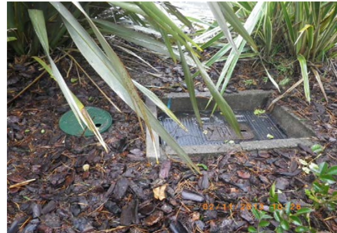
After the customers valve was installed.
