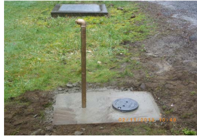
New blow off installed with the concrete poured.
