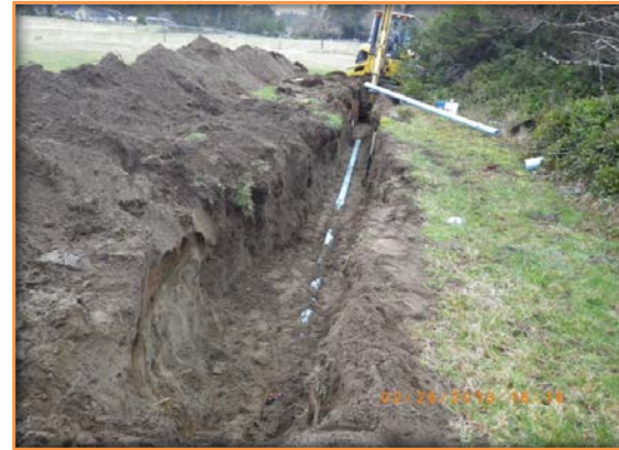
The start of Well # 2 Line replacement.
