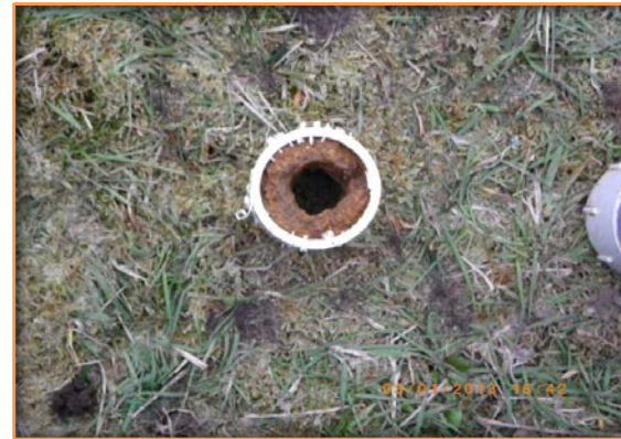
This is a picture of the inside of the old 2" line that was for Well # 2.
