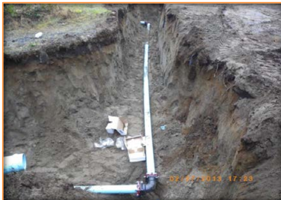
Picture of both 90s & the last stick of pipe installed.
