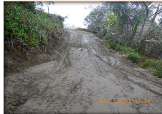
Looking up the hill after the pipe has been backfilled & before gravel.
