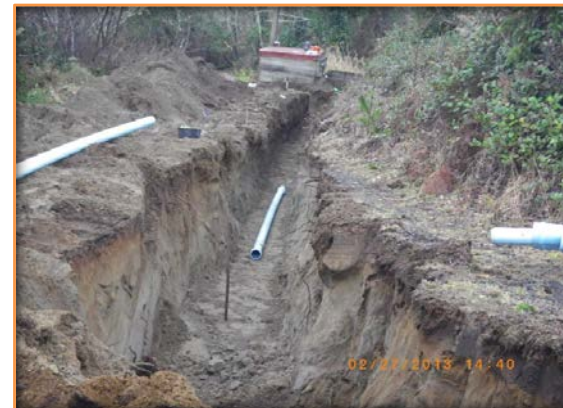
Picture of the new pipe coming up from the Well house.
