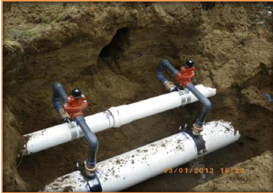
Picture of the two taps we made so we can flush the 6" & the new 4" line coming from Well # 2
