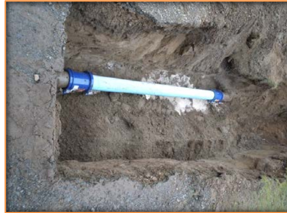
Main Break Repair on Bay Avenue
