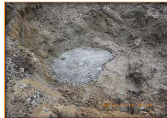
After one of the trust blocks were poured to help so the 90 doesn't blow apart from the pipe.
