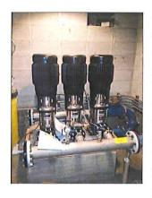
which included removing the existing pump and electrical system and replacing it with a package booster pump system. The new system includes three pumps and motors with variable frequency drives each sized to provide 85 gpm at 165 feet of total dynamic head. The package booster pump system is on a skid,
